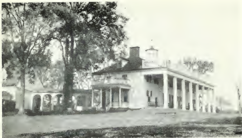
Mount Vernon, Showing Kitchen to the Left and Covered Way Leading to It
